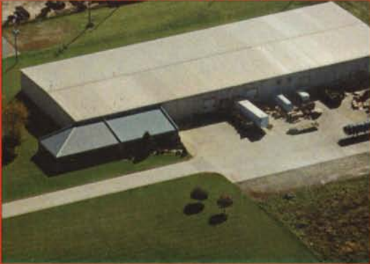
Excellent condition with room for expansion
